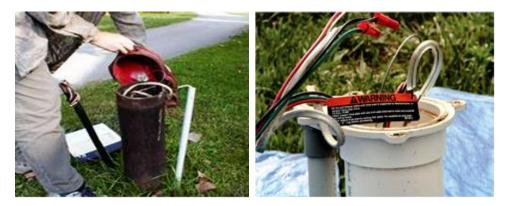
**Pour the 1 gallon of bleach directly into the well casing.** Rinse out the bottle with water and pour that water into the well casing.
